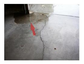
Figure 3: water entry into garage
