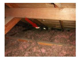
Figure 7: view of attic showing open vent
