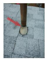
Figure 5: Sealant missing around roof vent
