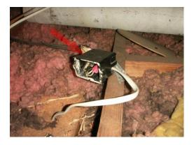
Figure 6: open electrical box near attic entrance
