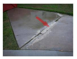
Figure 14: raised concrete at front driveway
