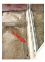
Figure 13: rear patio crack
