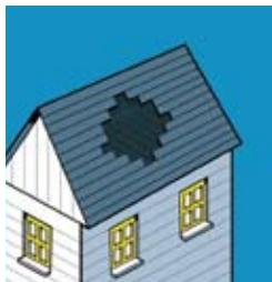
During a downpour, climb into the attic to look for leaking around chimneys, plumbing stacks, vents and skylights. Scan the underside of the sheathing for water stains.
